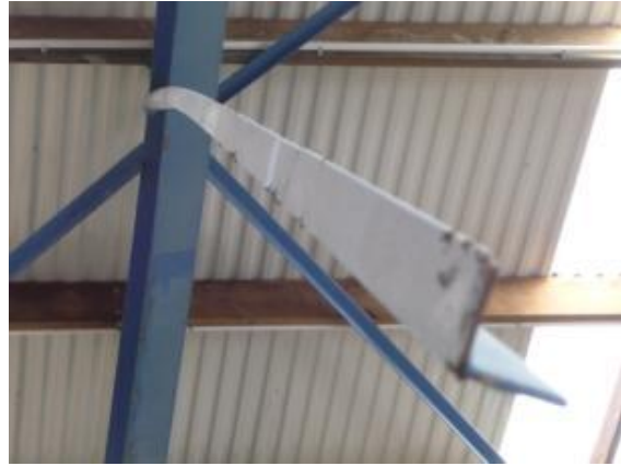
Figure 17: Industrial facility roof bracing From left to right ; (a) Global view, showing buckled brace and fractured brace; (b) Close –up view of fractures weld of tension brace. [Photos by M. Bruneau].
