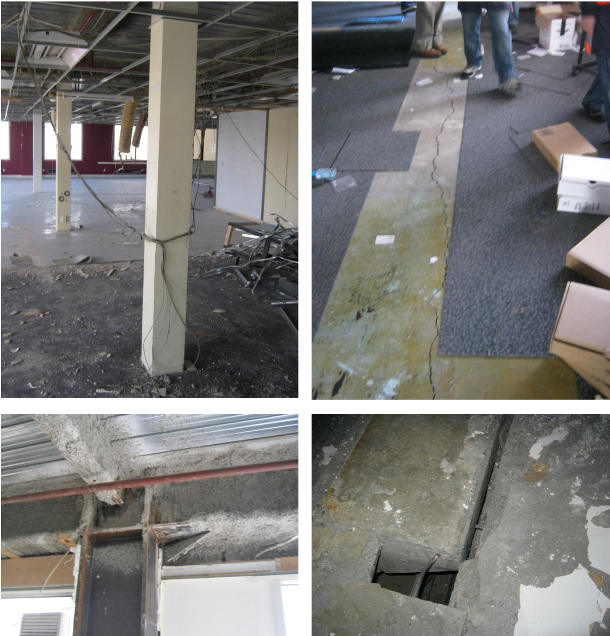
Figure 10: Seven storey PMRF building From top down and left to right:: (a) Internal view of partially stripped floor; (b) Crack in ground floor slab where perimeter (to the right of the crack) has moved downwards relative to the core; (c) Typical beam to column connection with fire protection partially removed for inspection; (d) Gap opening in stair at landing due to lateral movement (stairs had independent structural support). [Photos by C Clifton].
