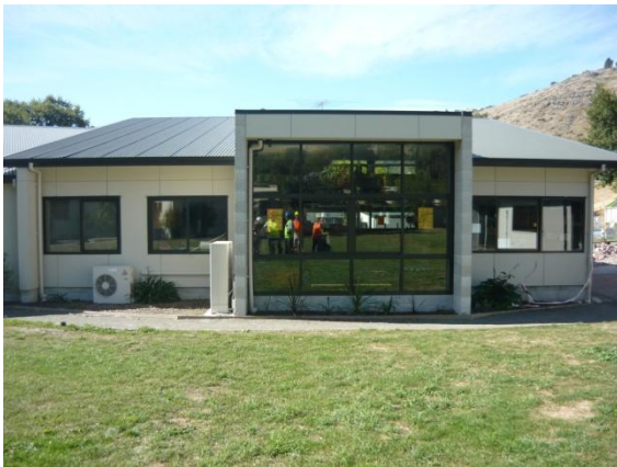
(a) Overall View from the South.
