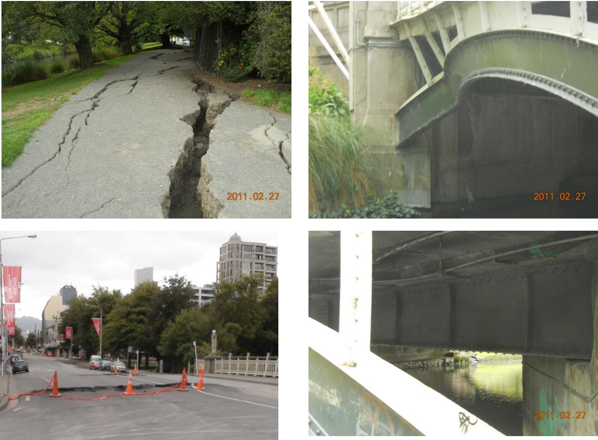
Figure 23: From top down and left to right: Colombo Street bridge (a) Slumping of riverbank close to bridge; (b) Buckling of fascia arches; (c) Slumping of abutments at end of bridge; (d) Undamaged straight riveted girders. [Photos by R Leon].
