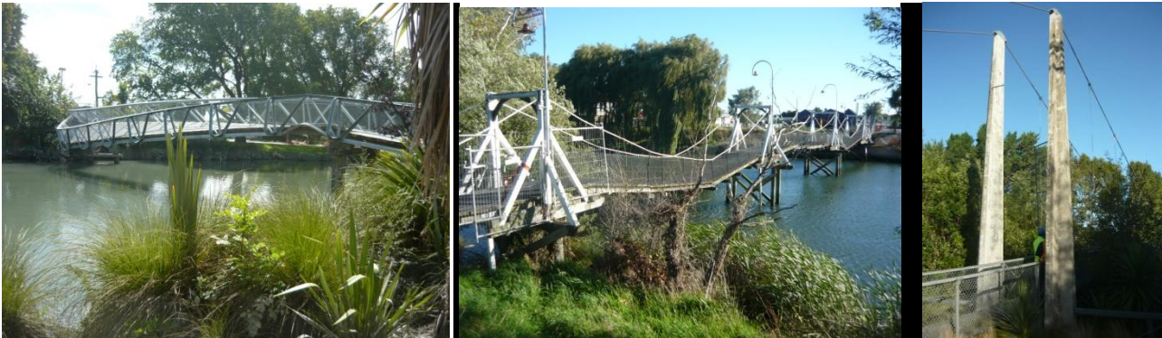
Figure 26: Footbridges; From top down and left to right: (a) Truss bridge over Avon River, (b) Suspension bridge with timber deck Over Kaiapoi river, (c) Suspension bridge at Groynes. [Photos by G MacRae].
