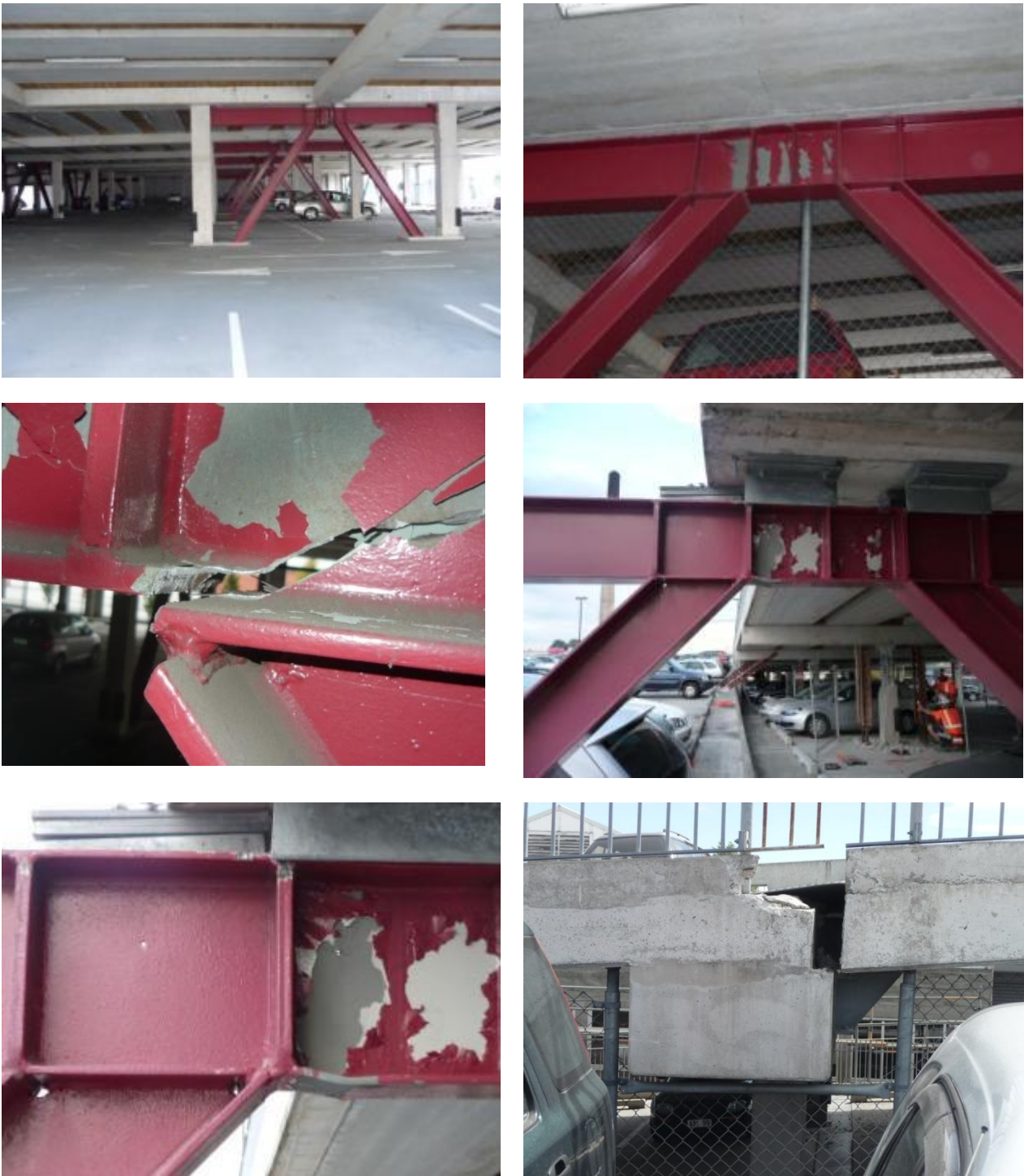
Figure 6: Parking garage on St Asaph St and Antigua St, Christchurch From top down and left to right: ; (a) Redundancy provided by multiple EBF bays; (b) Evidence of EBF link yielding; (c) Fractured link at lower level EBF; (d) Evidence of inelastic deformations at top level EBF; (e) Close-up view of same; (f) Displacement at expansion joint, top ramp. [Photos by M. Bruneau and C Clifton].
