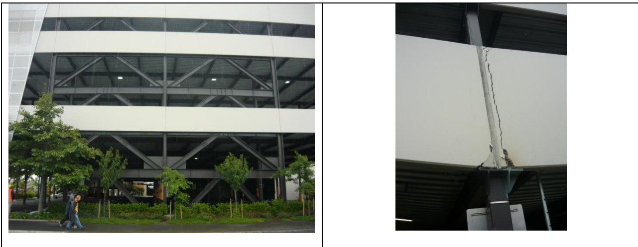
Figure 5: Shopping mall on Dilworth St and Clarence St, Christchurch From left to right; (a) View from the East, (b) Fracture of Precast Spandrel Beams on South side. [Photos by G. MacRae].
