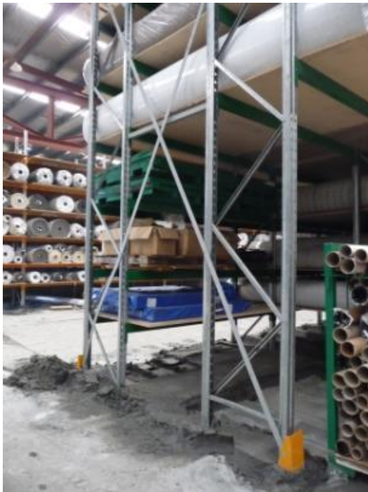
Figure 16: Industrial storage racks that survived, with evidence of soil liquefaction From left to right; (a) Global view; (b) Close -up of buckled brace. [Photos by M. Bruneau].
