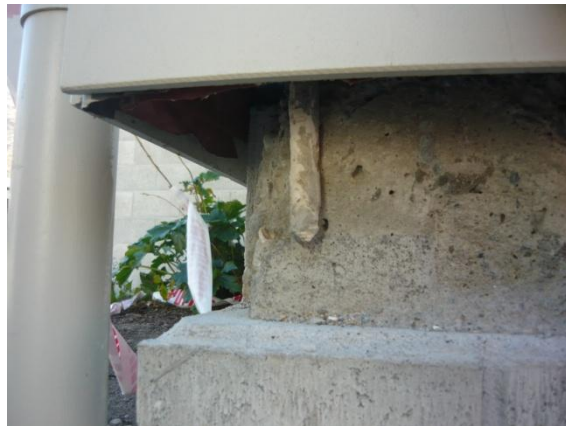
(b) Baseplate bolt at SE corner of the building.
