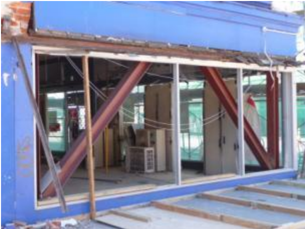
Figure 12 : Braced frame as a retrofit to unreinforced masonry building From left to right : (a) Close-up view; (b) Global view. [Photos by M. Bruneau and C Clifton].
