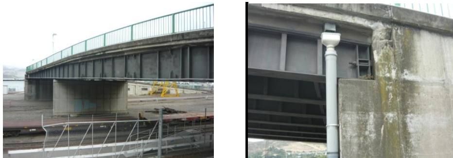
Figure 25: Lyttelton Port Bridge (a) Plate Girder (b) Abutment Spalling. [Photos by G MacRae].
