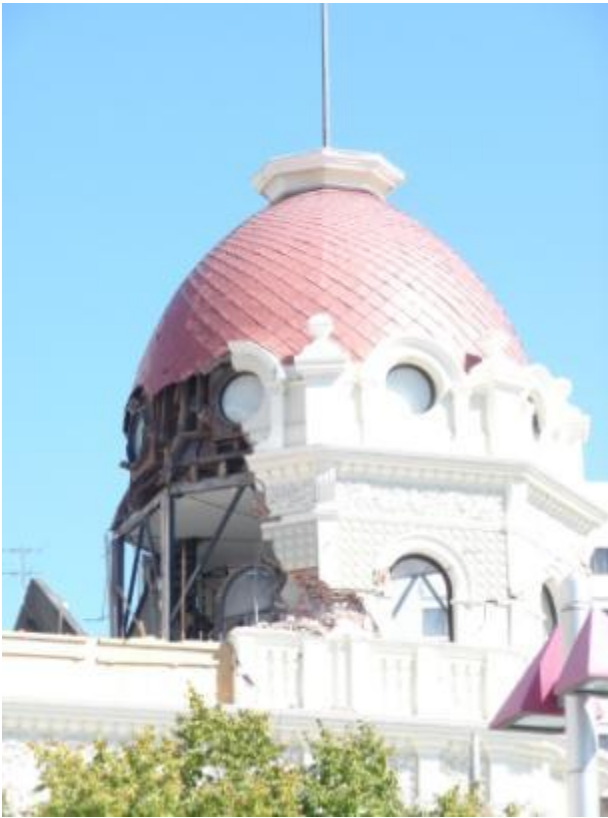
Figure 11: Braced dome at top of Regent on Worcester Building From left to right : (a) Global view; (b) Close-up view. [Photos by M. Bruneau].
