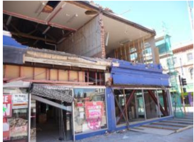
Figure 12 : Braced frame as a retrofit to unreinforced masonry building From left to right : (a) Close-up view; (b) Global view. [Photos by M. Bruneau and C Clifton].
