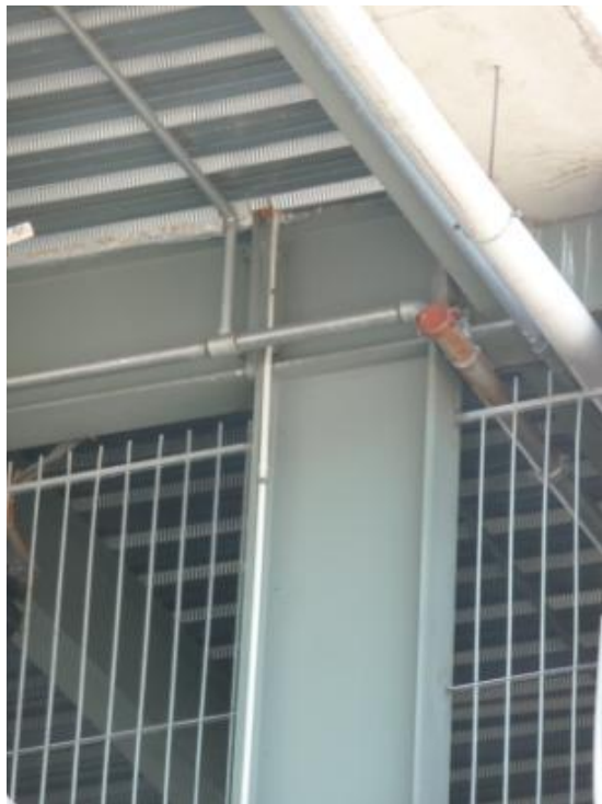
Figure 9: Low-rise MRF parking garage From top down and left to right:: (a) Global view; (b) and (c) Typical moment connections. [Photos by M. Bruneau].
