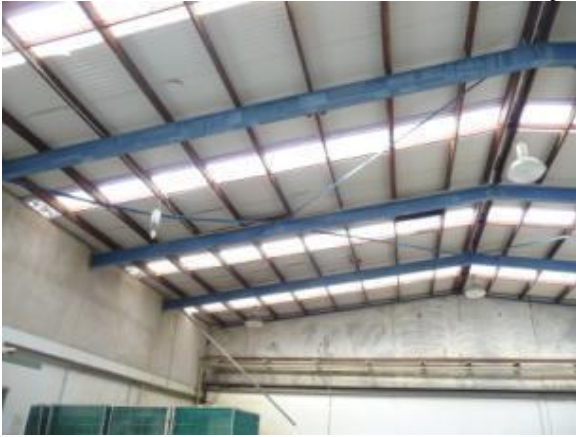
Figure 17: Industrial facility roof bracing From left to right ; (a) Global view, showing buckled brace and fractured brace; (b) Close –up view of fractures weld of tension brace. [Photos by M. Bruneau].
