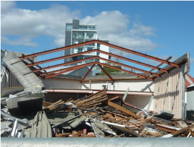
Figure 19: Failure of roof and walls in older industrial facility on Salisbury Street. [Photo by G MacRae].
