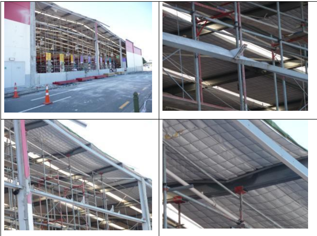
Figure 18 : Failure of tilt-up panel connections From top down and left to right: (a) Global view; (b) Close –up view of fractures connection; (c) Global view of buckled beams; (d) Local view of one such beam. [Photos by M. Bruneau].
