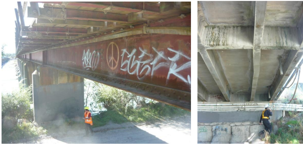
Figure 24: Waimakariri Bridges, South end (a) Old Rail Bridge, (b) Old road bridge. [Photos by G MacRae].
